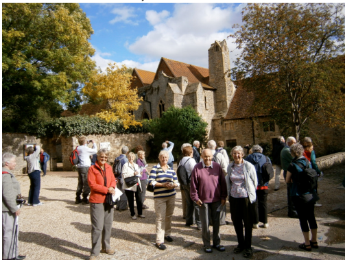
Gathering in front of Abingdon's unique chimney
